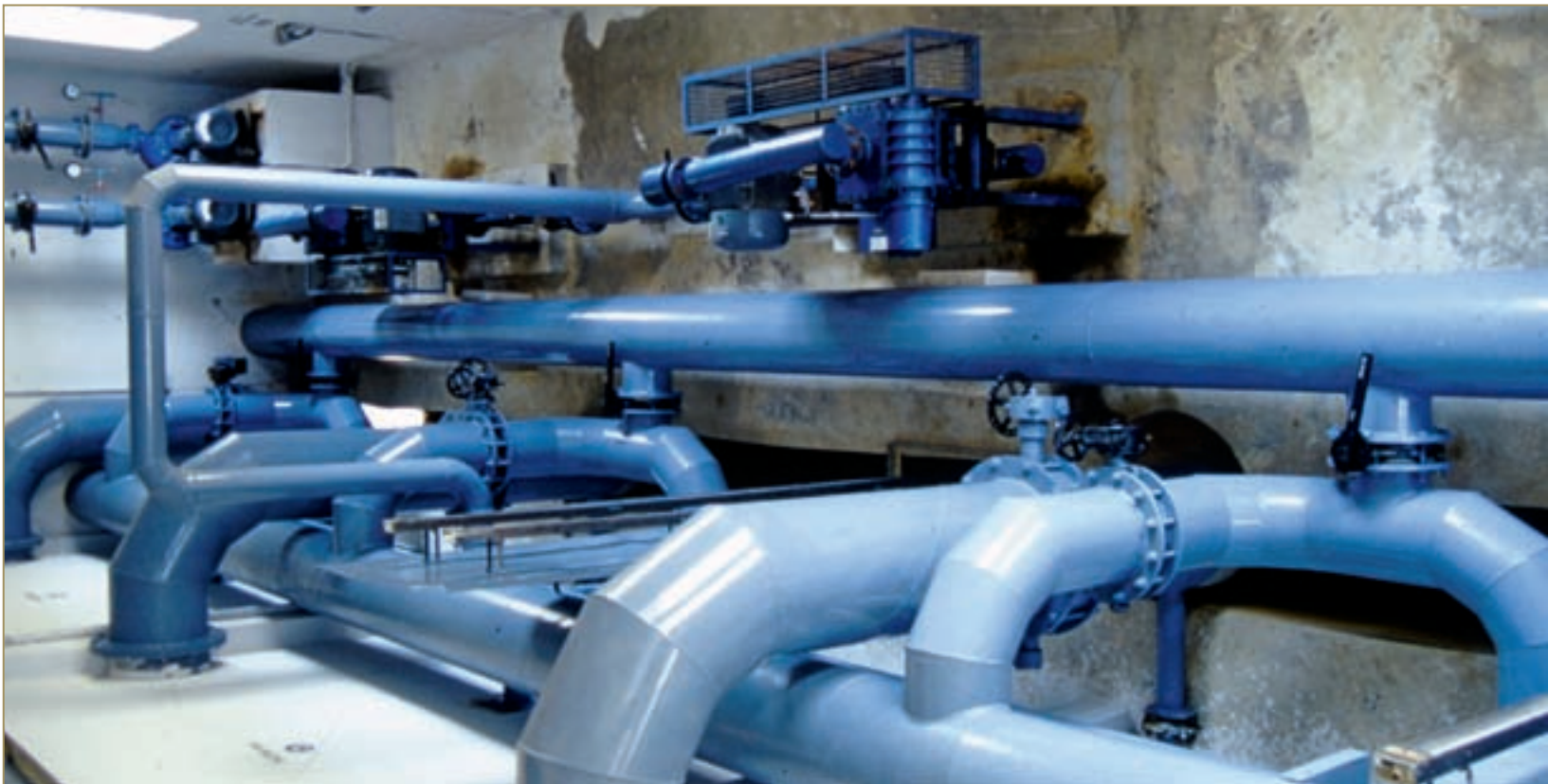
Following that, the water is passed through a series of sand filters and then chlorinated before distribution. Pictures (a), (b) and (c) show views of the pump house.
