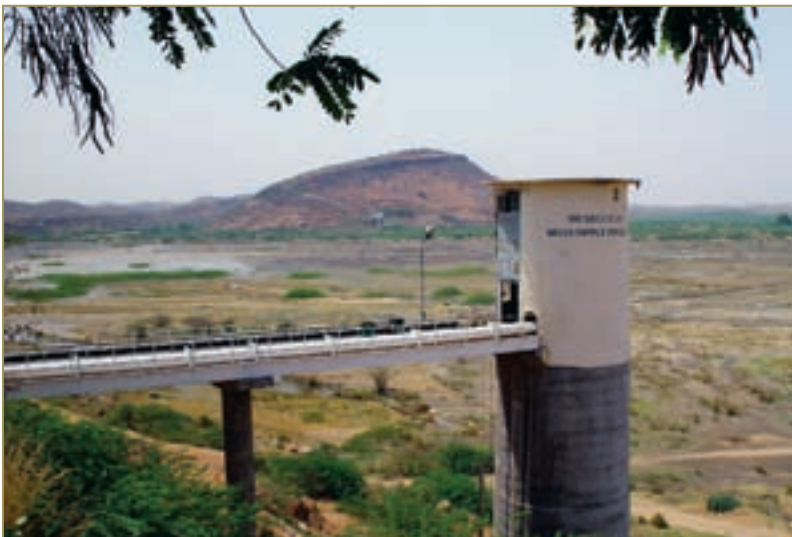
The collection well where a pump pulls the water from all the infiltration wells and sends it further for distribution.
