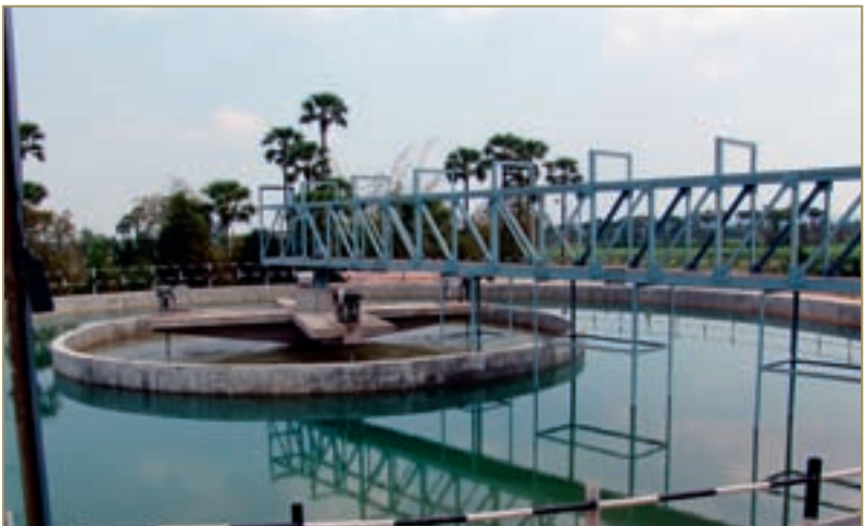
Sediments are then removed by stirring the water using a clariflocculator.
