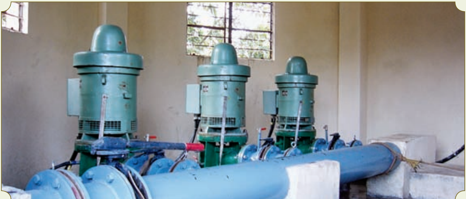
Suction pumps inside the intake well.
