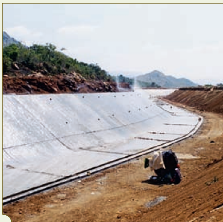
Cement lining of the canal in progress.
