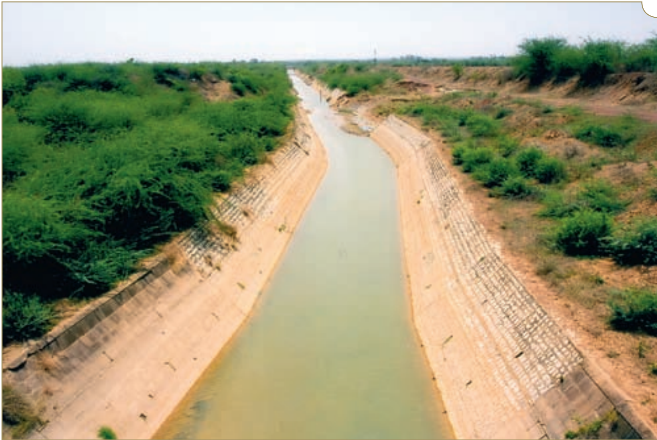
Two views of a section of the canal on the Tamil Nadu side before (top) and after (below) renovation. An essential feature of the renovation is that mud from the sides of the canal is prevented from being washed down by rain. This picture shows an upstream view.
