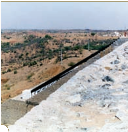
Pipe carrying water brought down to ground level and taken to the pump house, which is seen clearly in the picture on the right.
