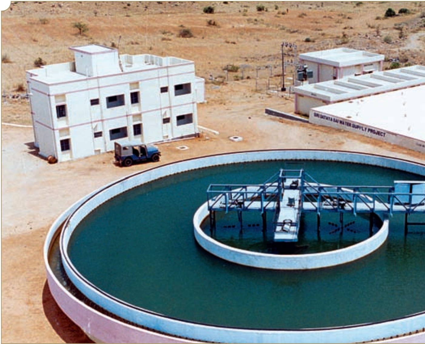
This circular tank in the foreground is used for precipitating out solid contaminants. This is done by adding a suitable solvent and stirring the water using the long arm seen in the picture. This is one of the many processes involved in the purification of the water before it is distributed. Additional purification using sand filters is done in the building on the left, near which a truck is parked.
