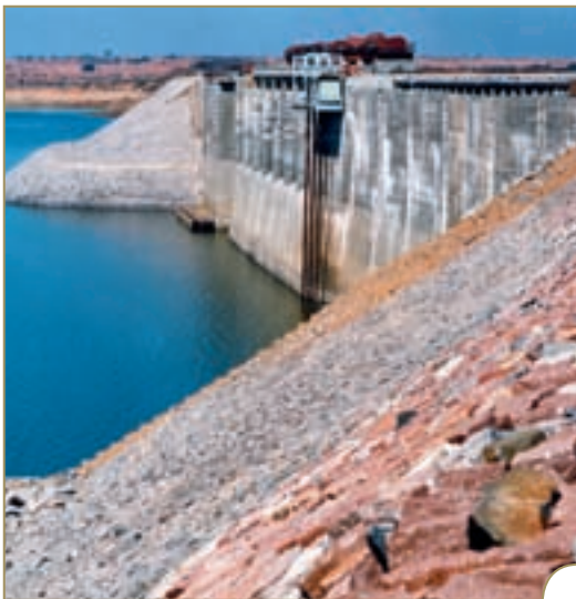
Water being drawn from an irrigation dam by three vertical pipes.
