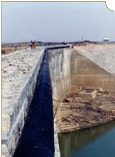
The water drawn is taken by the pipe seen above, along the wall of the dam and later brought to the ground level.
