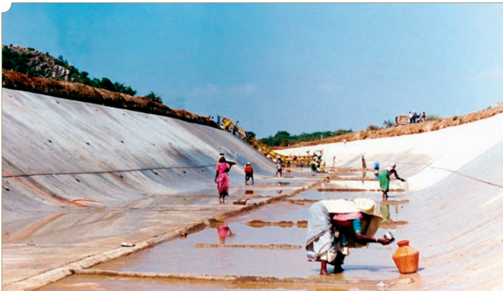
Curing of the cement lining is in progress.
