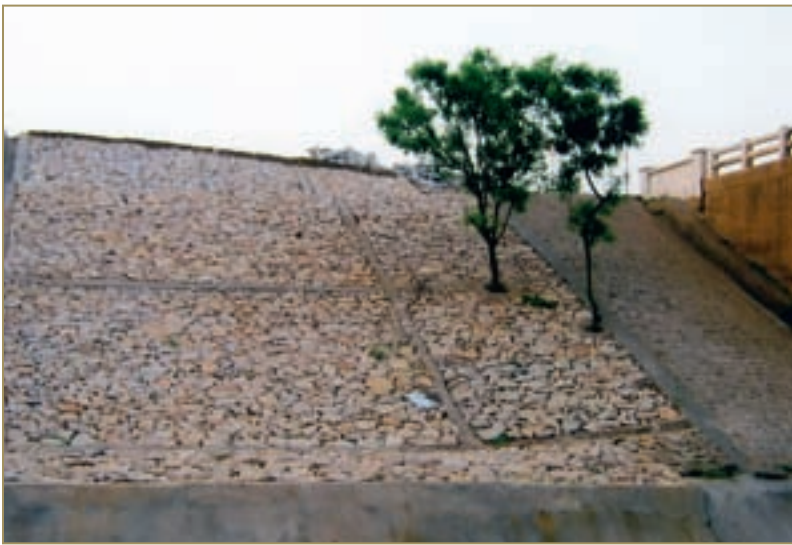
The two pictures above highlight once more how the slopes on the side of the canal have been taken care of, to prevent soil erosion and the consequent choking of the canal.
