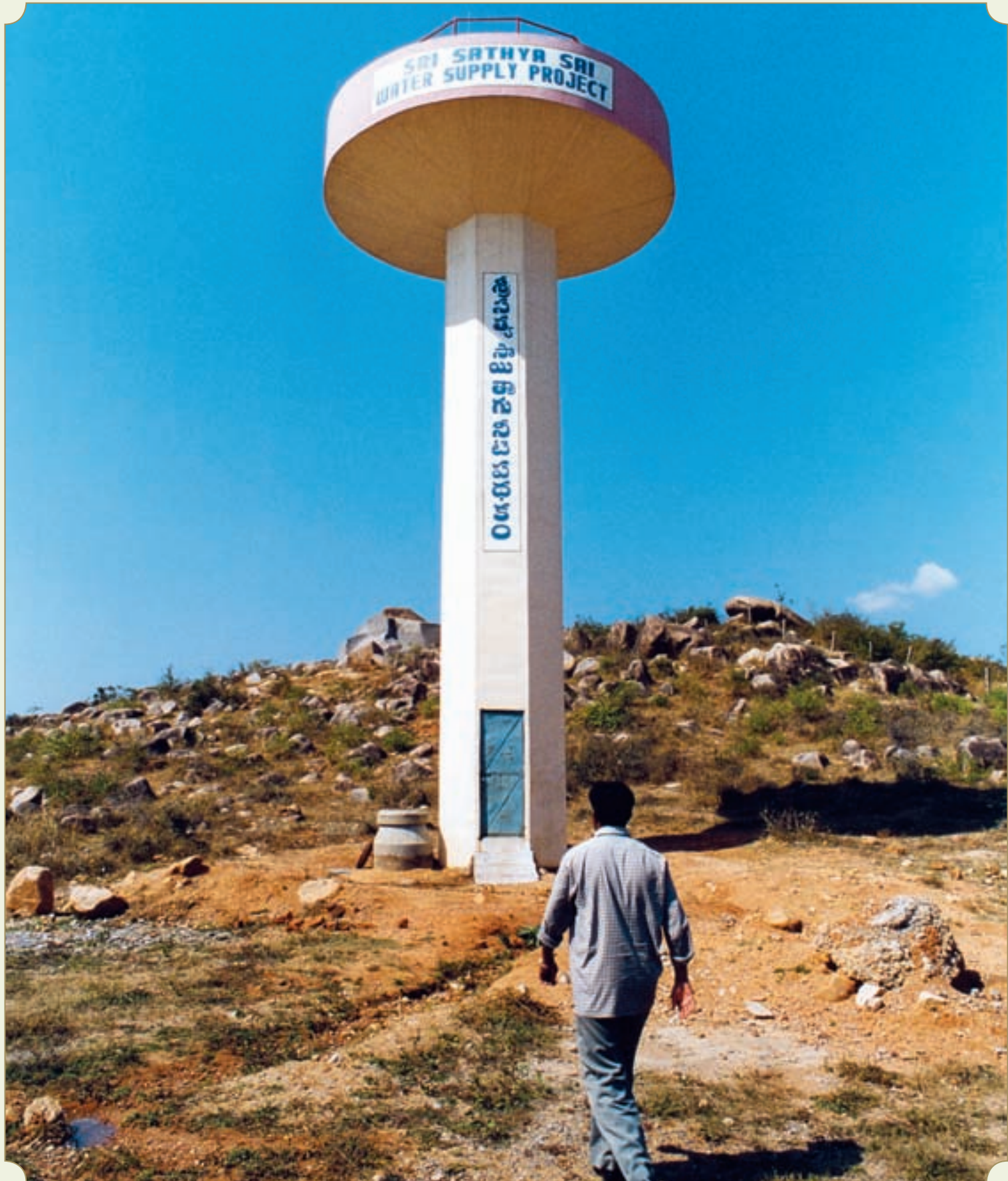
Another storage tank. This one is not as tall but is placed in a slightly elevated spot to take advantage of gravity.
