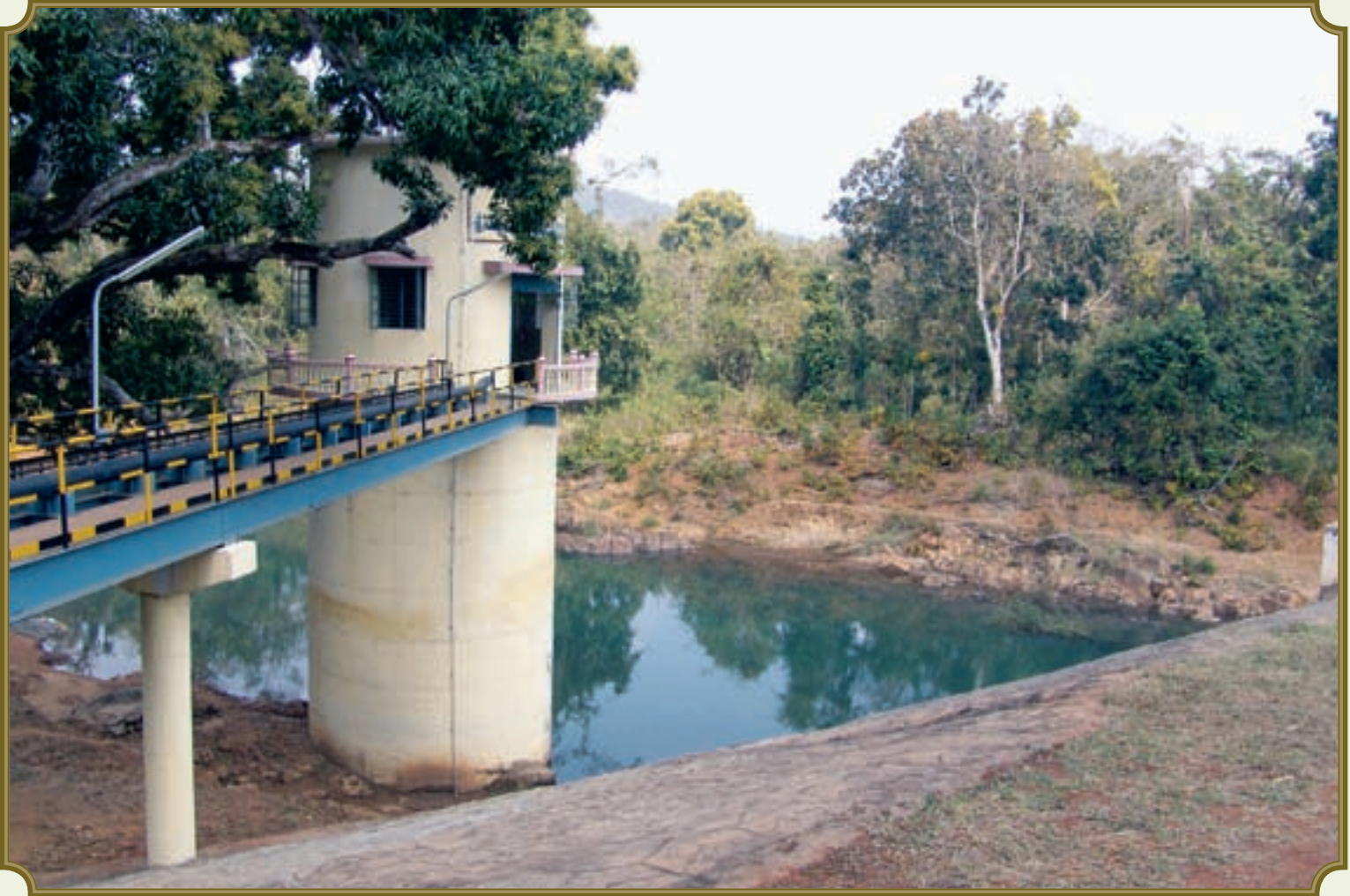
Intake well located on the mountain stream, after completion.
