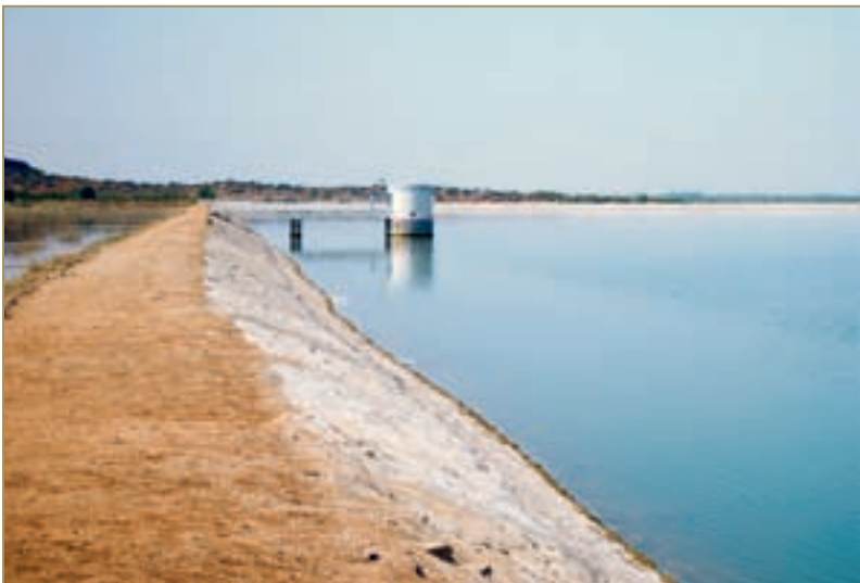
A portion of the Anantapur tank where the intake well is located. A pump here draws water from the tank and sends it to a purification plant, from which it is distributed.
