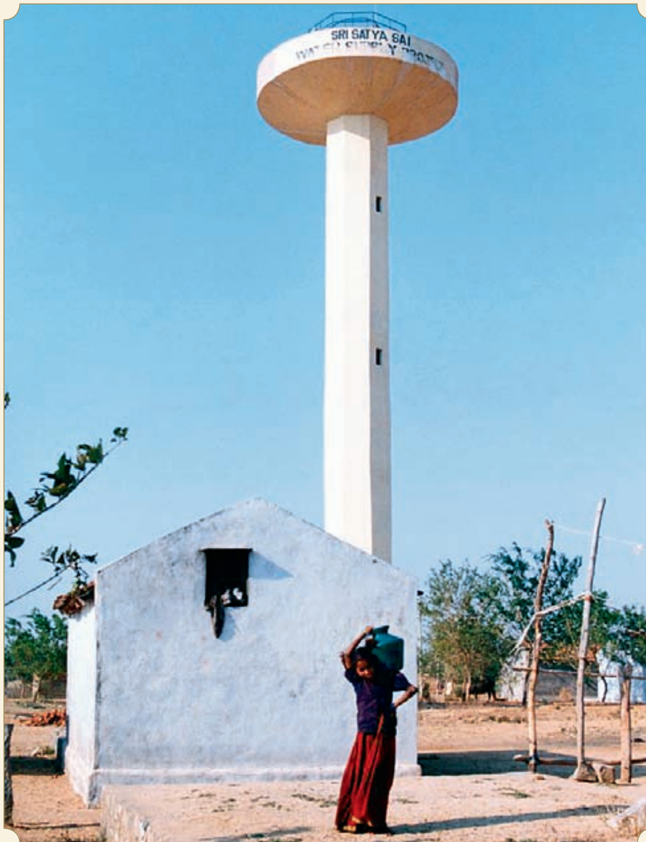
Unlike in Anantapur District, the terrain in the northern districts is relatively flat. There was thus no need to pump the water up and down while transporting it over distances. Instead, tall storage tanks were built, which, using gravity flow, could supply water to many villages. Shown here is one such tank.
