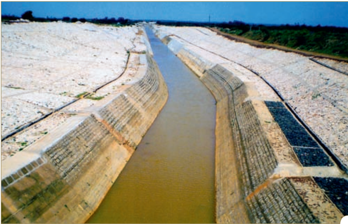
Two views of a section of the canal on the Tamil Nadu side before (top) and after (below) renovation. An essential feature of the renovation is that mud from the sides of the canal is prevented from being washed down by rain. This picture shows an upstream view.
