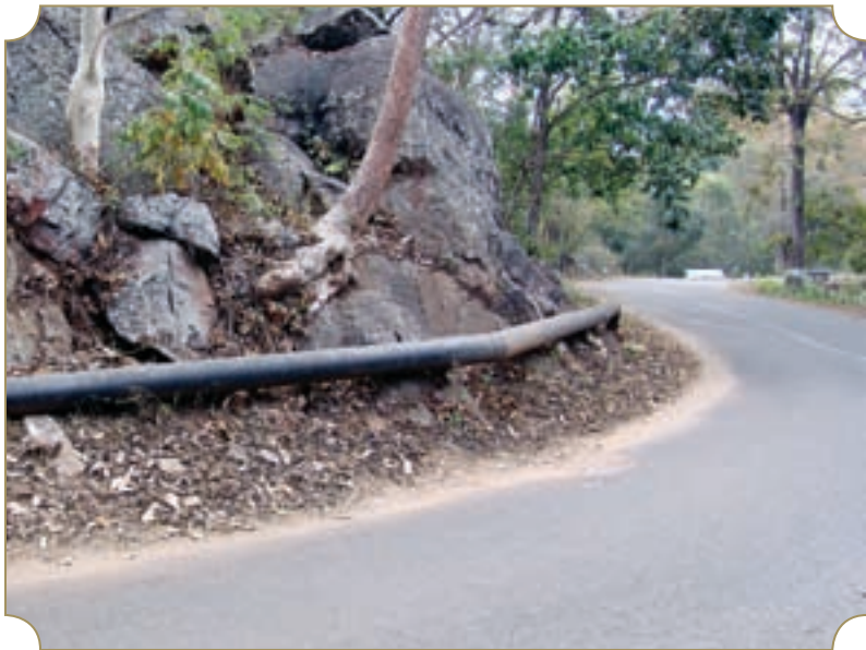
The picture above shows how pipes were laid close to the road whenever possible. This was mandatory.
