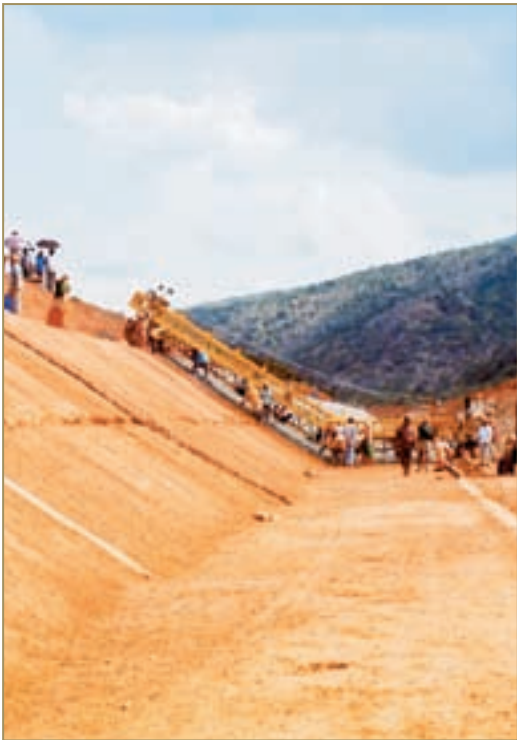
Canal renovation in progress. Before the canal was lined with cement, the seepage prevention film was introduced at the bottom of the canal and on both sides.
