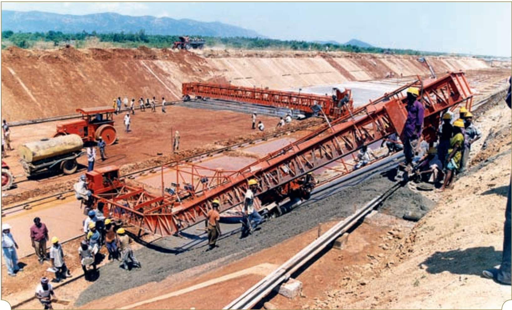
The two pictures on the top show renovation work in progress in the mountain section. In some places, the canal is very wide since it caters to irrigation work in that region. The picture below shows how the cementing work was done using machines that lined the bottom and the sides simultaneously.
