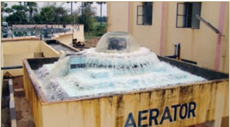
Incoming water is first aerated as shown above.
