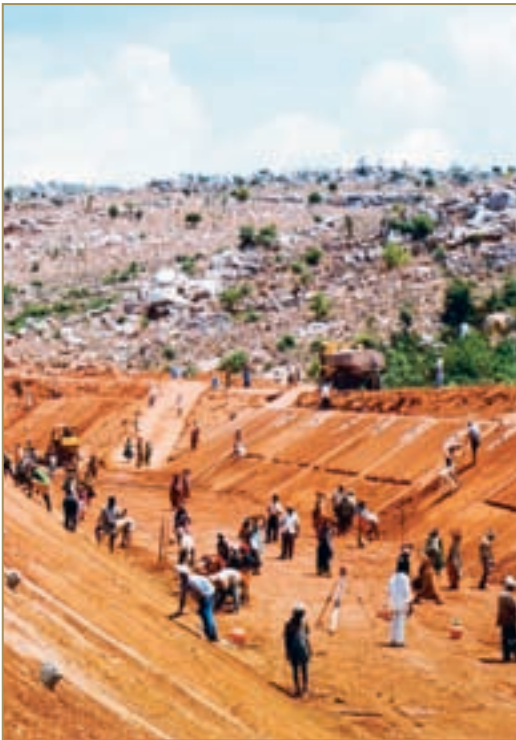
Canal renovation in progress. Before the canal was lined with cement, the seepage prevention film was introduced at the bottom of the canal and on both sides.
