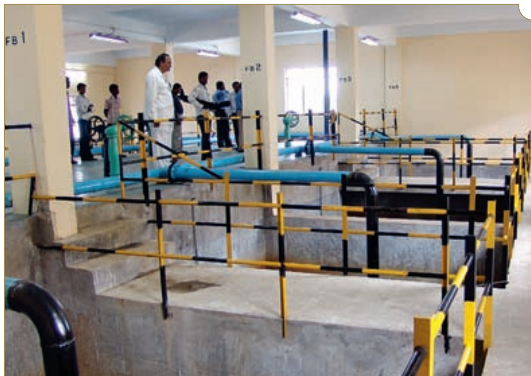
After aeration, the water is then purified through a series of sand filters, after which it is chlorinated before distribution.
