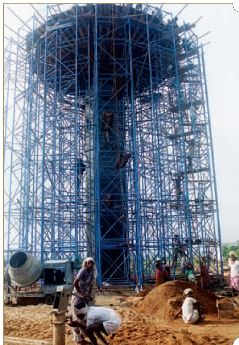
An overhead reservoir under construction.
