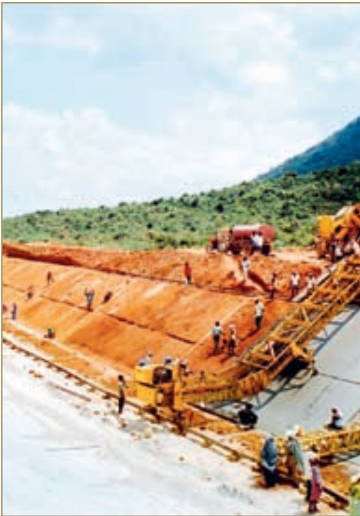
Canal renovation in progress. Before the canal was lined with cement, the seepage prevention film was introduced at the bottom of the canal and on both sides.
