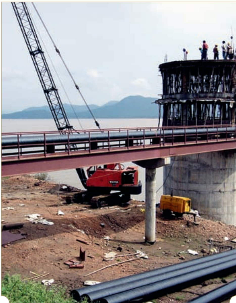
Pictures of collection wells located on the river, under construction. There are two such wells, one on each bank.
