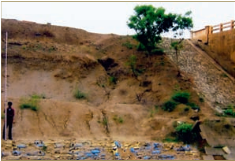
The two pictures above highlight once more how the slopes on the side of the canal have been taken care of, to prevent soil erosion and the consequent choking of the canal.
