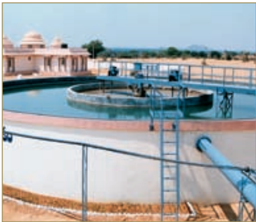
The solid deposits are then removed using a clarifloculator.
