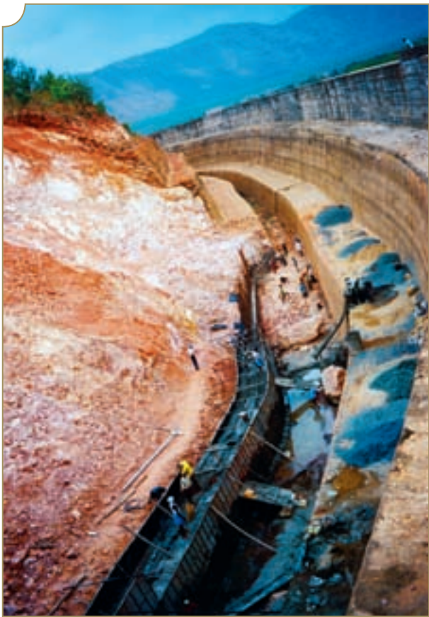
The two pictures on the top show renovation work in progress in the mountain section. In some places, the canal is very wide since it caters to irrigation work in that region. The picture below shows how the cementing work was done using machines that lined the bottom and the sides simultaneously.
