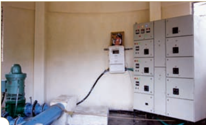
Seen above is one of the two completed collection wells and some inside views showing the pumps and the switchboard. Water is sent from here to the pump house for filtration and purification.
