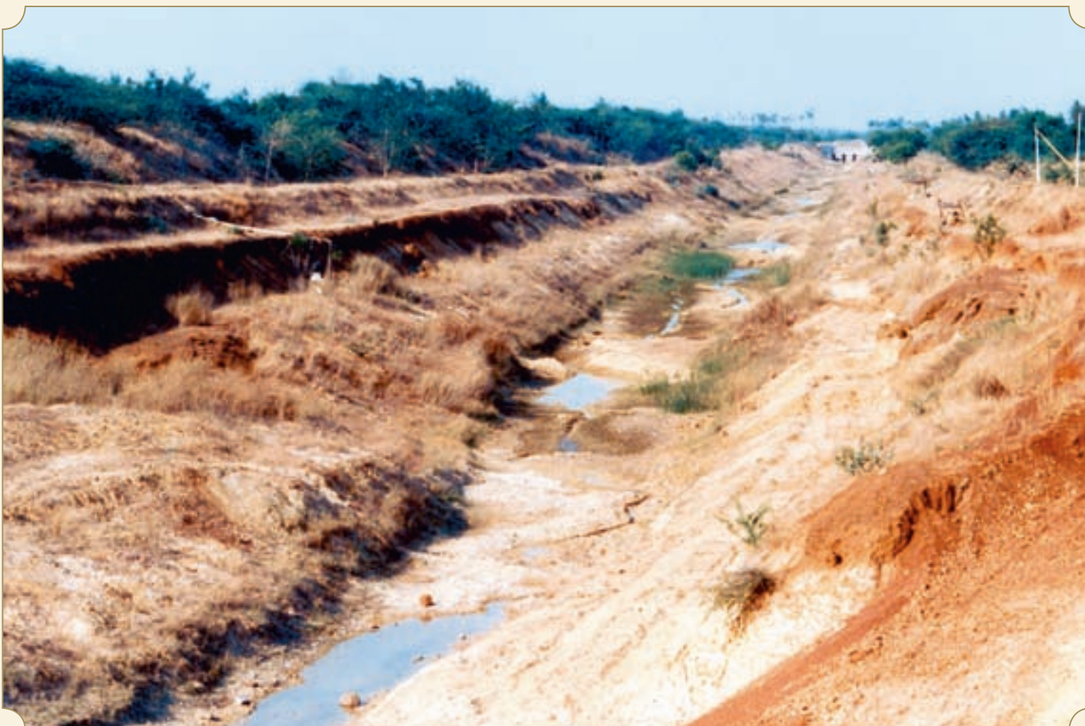
A view of the canal near the Andhra Pradesh-Tamil Nadu border. The poor quality of the canal construction is clearly evident.
