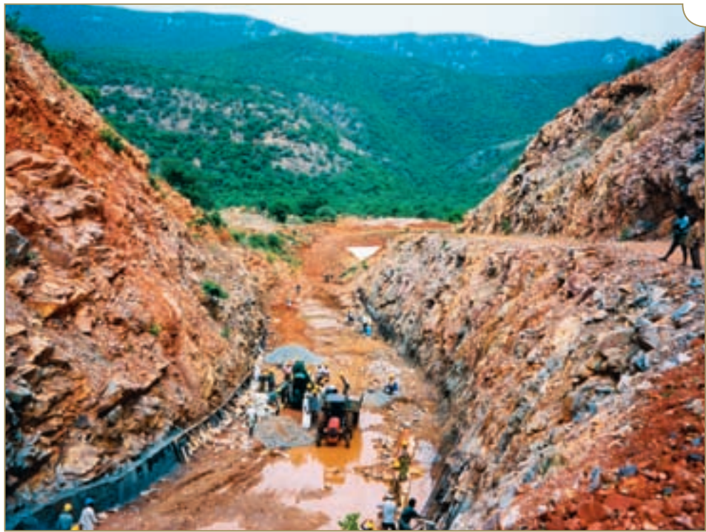
The two pictures on the top show renovation work in progress in the mountain section. In some places, the canal is very wide since it caters to irrigation work in that region. The picture below shows how the cementing work was done using machines that lined the bottom and the sides simultaneously.
