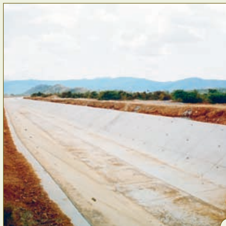
Cement lining completed.
